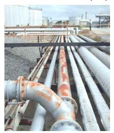
possible breach that might contribute to Corrosion Under Insulation (CUI). Using API-570 guidelines and experience, InterSpec is able to inspect insulated piping with minimal removal
